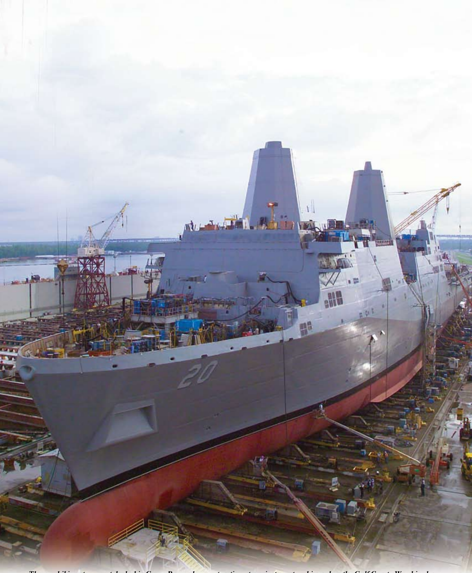
The amphibious transport dock ship Green Bay under construction at a private-sector shipyard on the Gulf Coast. Warships have become much more complex as a result of the information revolution, requiring support and sustainment skills that often can be obtained more affordably in the private sector than through traditional, public-sector channels. (Image: Huntington Ingalls Industries)
