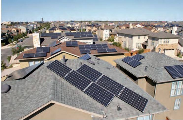
Solar power is one type of distributed energy resource that is dependent on weather conditions, making it challenging for operators to match generation load at every moment.
